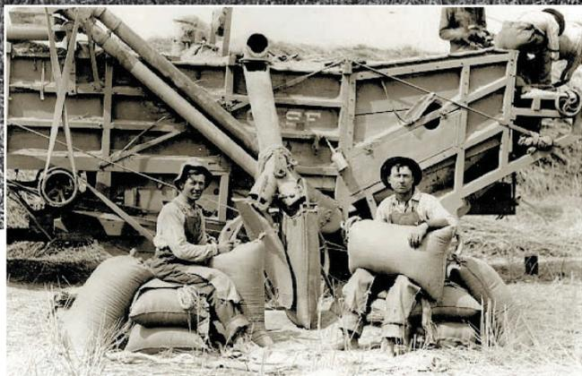
Machines that both reaped (cut) and threshed (separated the wheat from the shaft) were called combines. They were widely used by the 1890s. Some required as many as forty-four horses. Later, self-propelled steam combines were used in the Palouse region.
