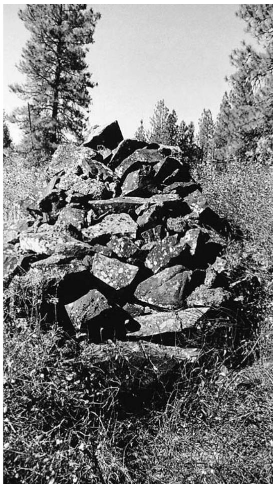
This pile of basalt rocks is actually an oven. Italian railroad construction crews in eastern Washington made the ovens to bake their bread.
