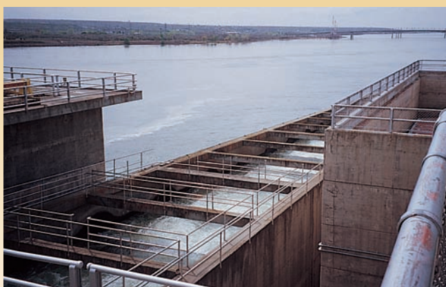
McNary Dam, like others on the lower Columbia and Snake Rivers, have fish ladders to help fish get back to their spawning grounds. Photos by Mike Green
