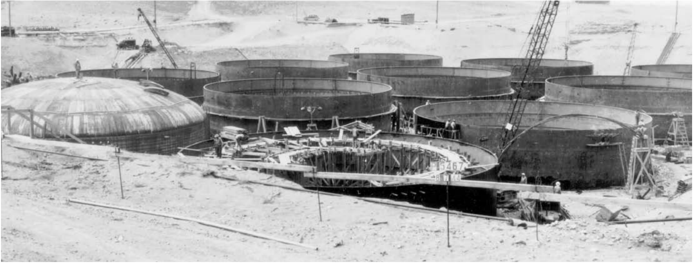
Hanford nuclear waste storage tanks are under construction. Double-wall steel storage tanks have been built to replace some of the leaking ones. Eventually, some of the wastes will be pumped out and contained in safe glass logs at a plant that has yet to be built. To get a sense of size, note the workers in the photo. Photo courtesy of Columbia River Exhibition
