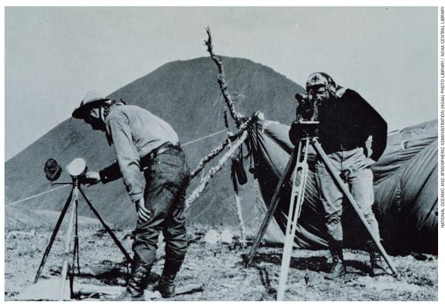
This heliograph used mirrors to reflect light from the Sun to signal messages over long distances. The user tapped out a message using a key check attached to the mirror. His partner looked for the return message.
